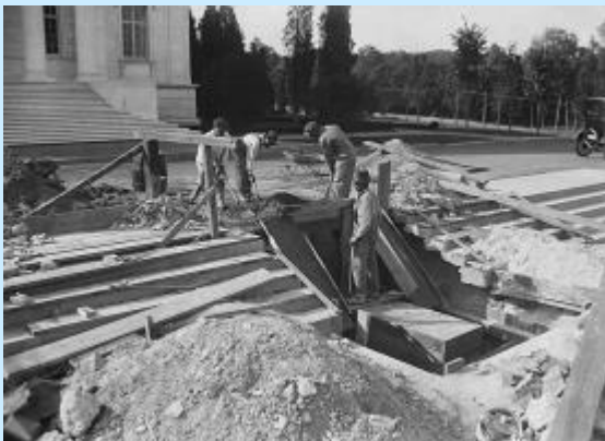
Construction begins on the Tomb of the Unknown Soldier, 1921
